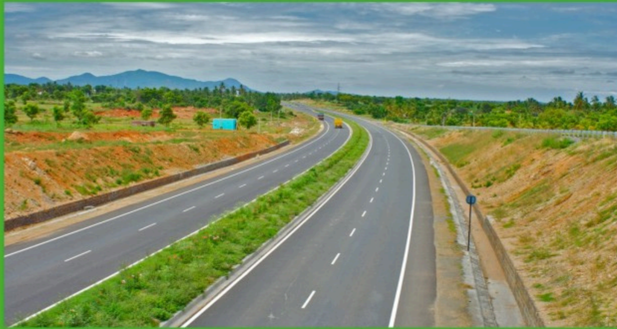
Nagpur - Amravati - Mumbai Express Highway NH6
